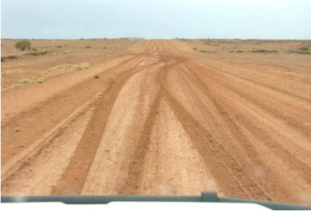
Picture 73: Even an easy gravel road can become dangerous with rain
